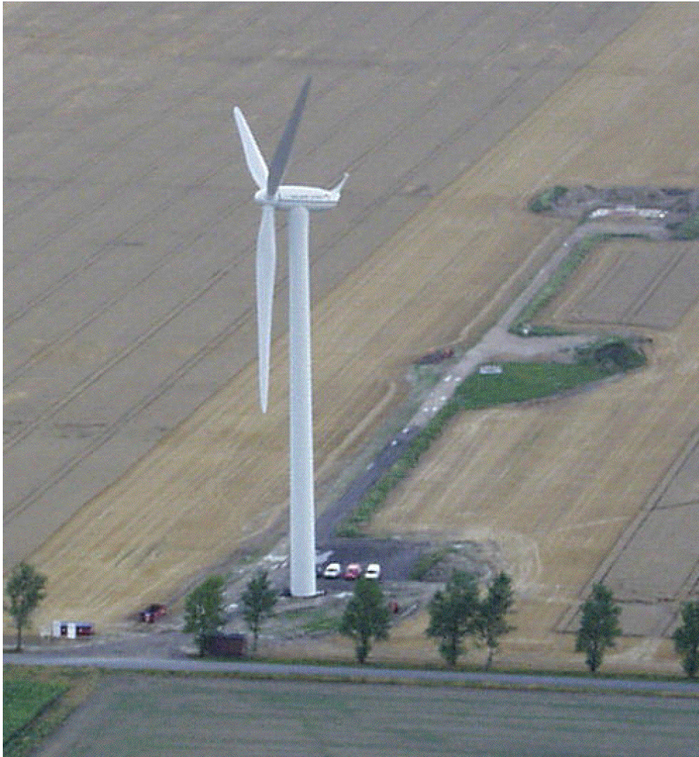
Figure 9. A 2 MW turbine with a 72 m rotor diameter on a 68 m tower. [www.windpower.dk]
